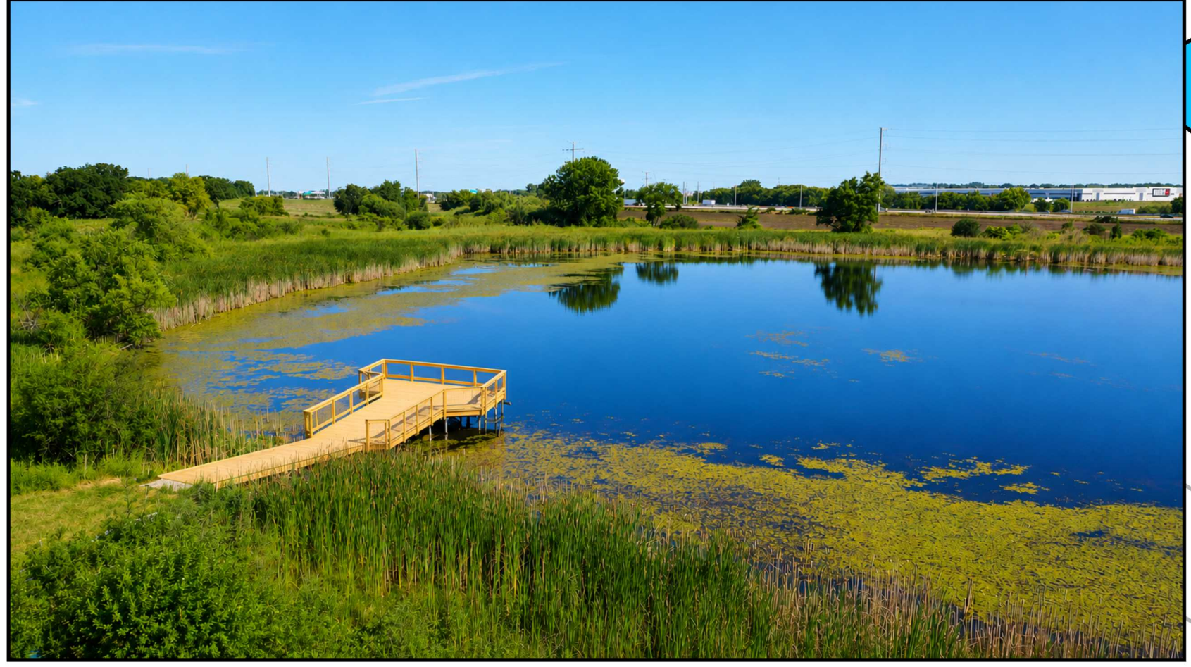
New Fishing Pier and Stone Outcropping Areas
